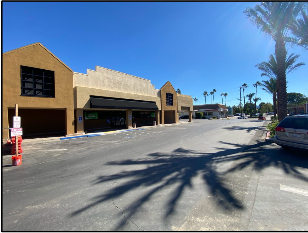
21) View of the storefronts and veterinary office on the Subject Property, southeast-facing from the parking lot.
