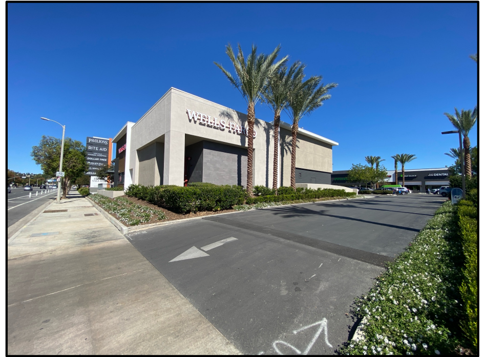
24) View of the bank on the west side of the Subject Property, northeast-facing from Platt Avenue.
