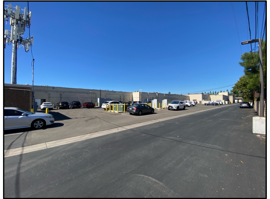
16) View of the rear of the shopping center on the Subject Property, northwest-facing.
