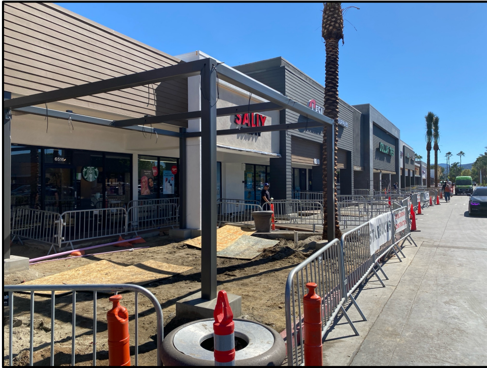
19) View of the storefronts and current construction (renovations) on the Subject Property, southeast-facing from the parking lot.
