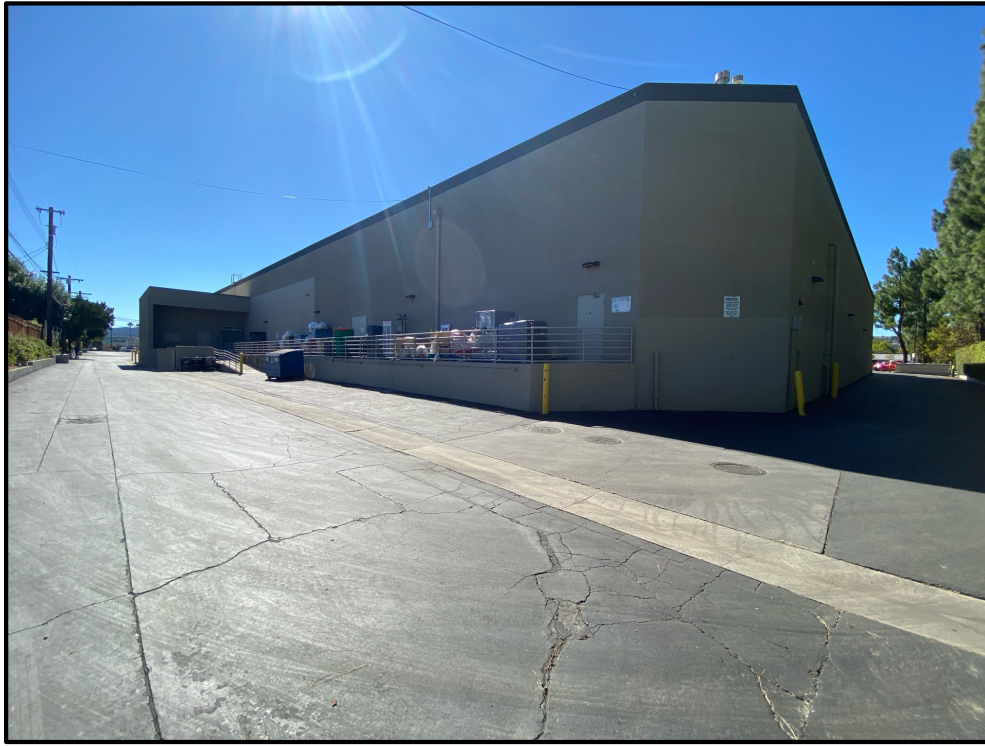
17) View of the northeast corner of the shopping center on the Subject Property, southwest-facing.
