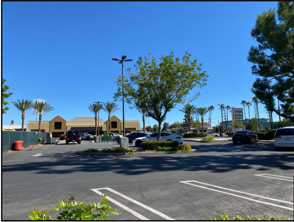
3) View of the Subject Property, east-facing from Platt Avenue.
