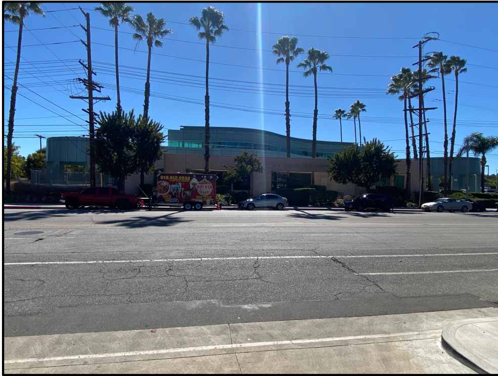
27) View of the library across the street to the south of the Subject Property, south-facing from Victory Boulevard.
