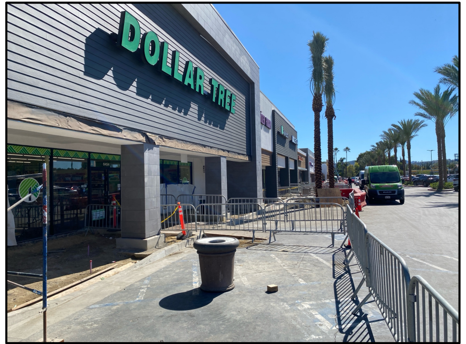
20) View of the storefronts and current construction (renovations) on the Subject Property, southeast-facing from the parking lot.
