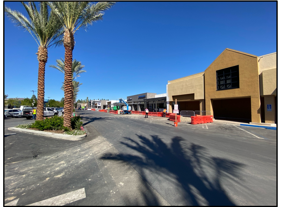
22) View of the storefronts and current construction (renovations) on the Subject Property, northeast-facing from the parking lot.
