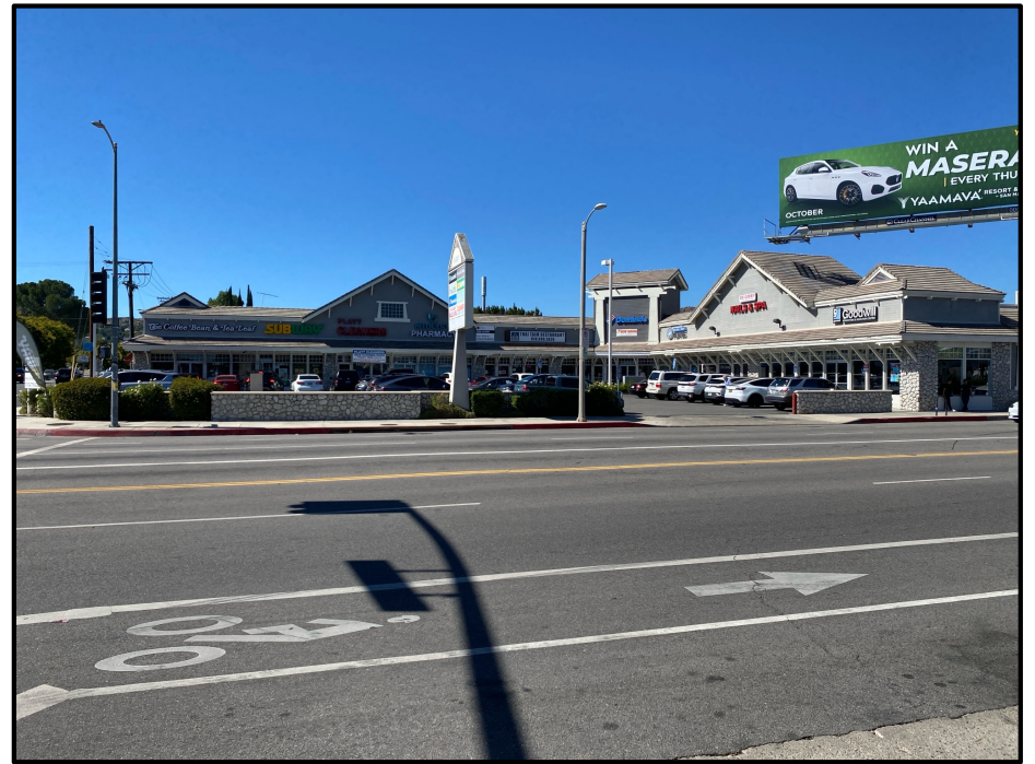
30) View of the commercial property across the street to the west of the Subject Property, west-facing from Platt Avenue.
