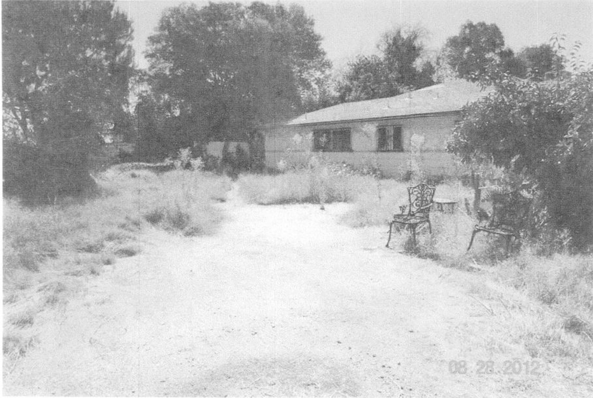
Exterior - Before (August 28, 2012)
